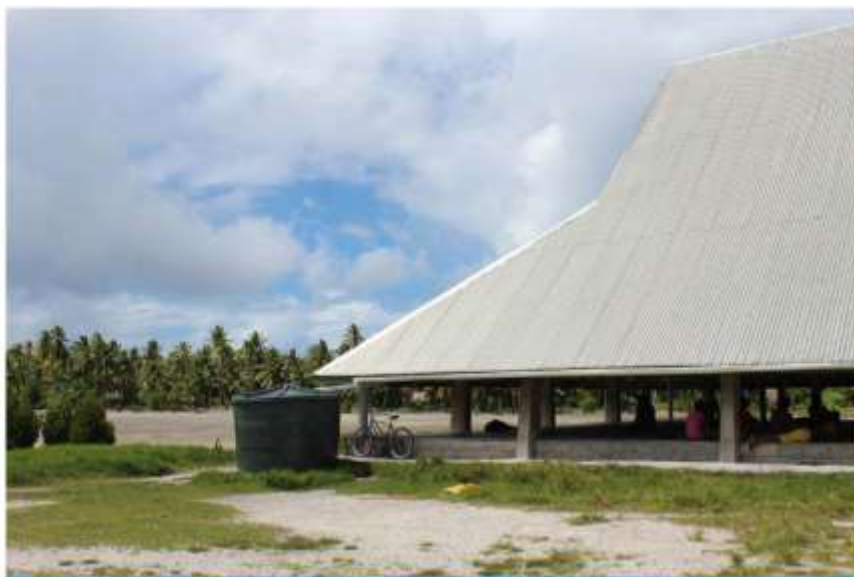
Zbieranie deszczówki z dachu, fot. Department of Foreign Affairs and Trade, CC BY 2.0
